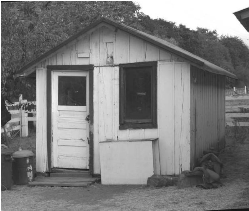
Cottage near entry to stables viewed from the north
