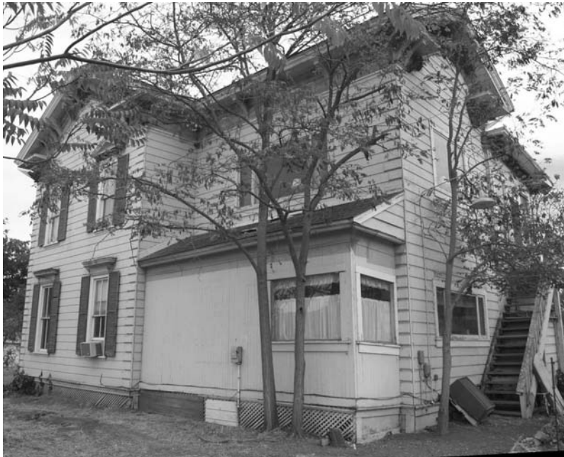
Northwest corner of Bailey/Fellows House
