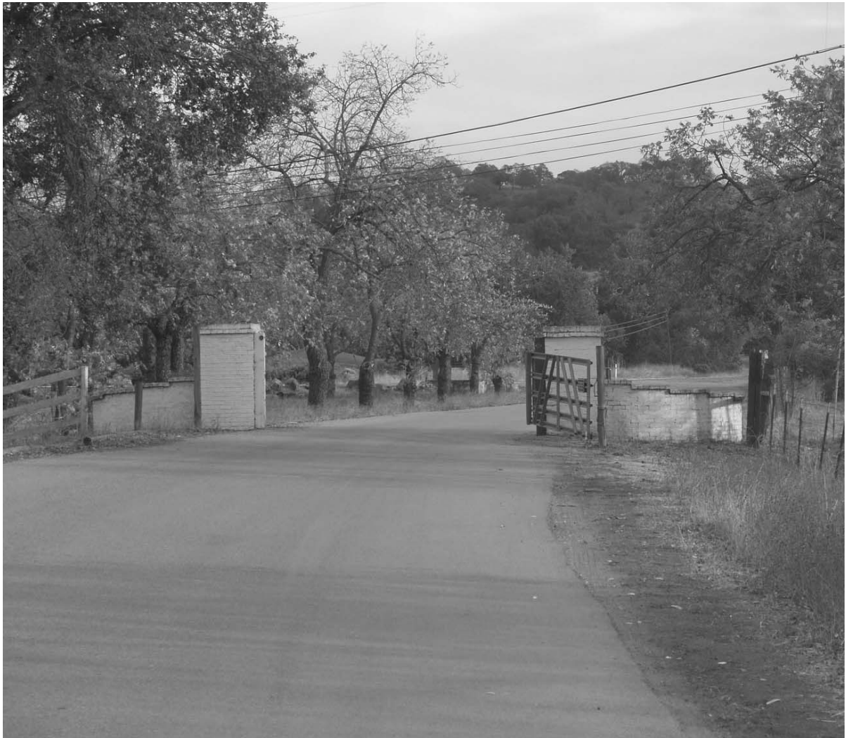
Entry gates and pillars viewed from the north
