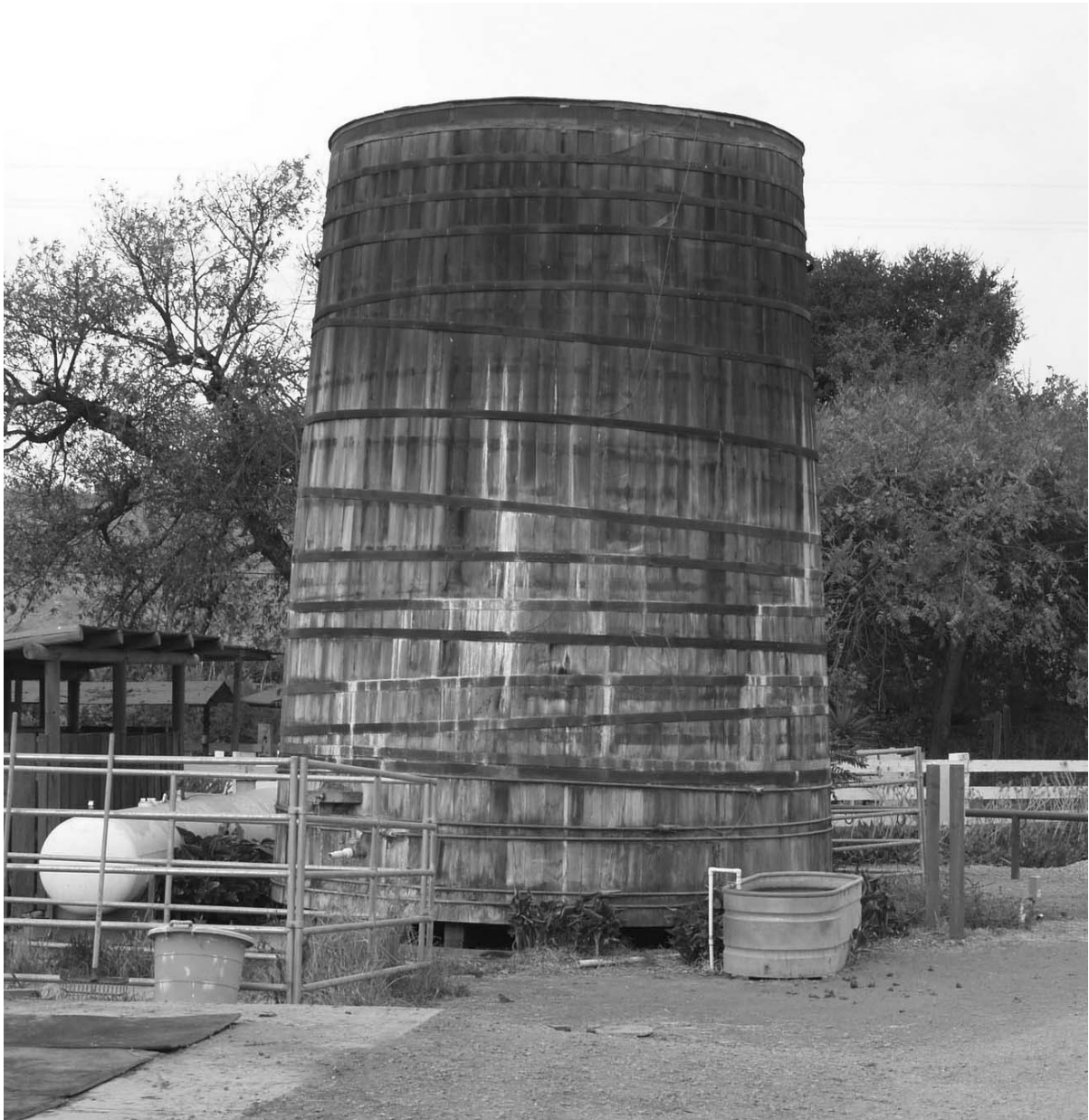
Water tank near entry to stables viewed from the west
