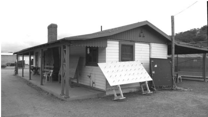
Office building viewed from the northeast
