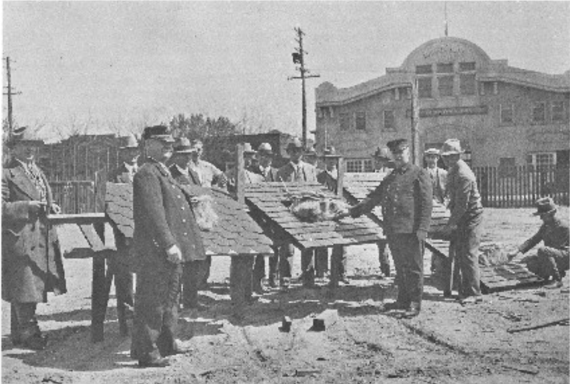
The fire-retarding qualities of composition roofing are demonstrated, about 1930, in a vacant lot off Bart Santa Clara Street near 4th. Fire officers are (left) veterans Captain John Gilman, acting Fire Marshal, and Chief Charles Plummer.
