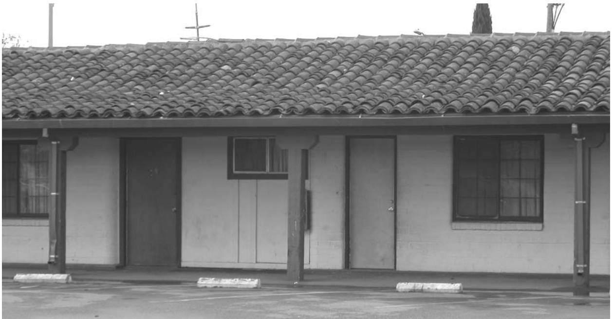
View of south wing from the north. Note middle unit with high window at what was originally a carport. 04/03
