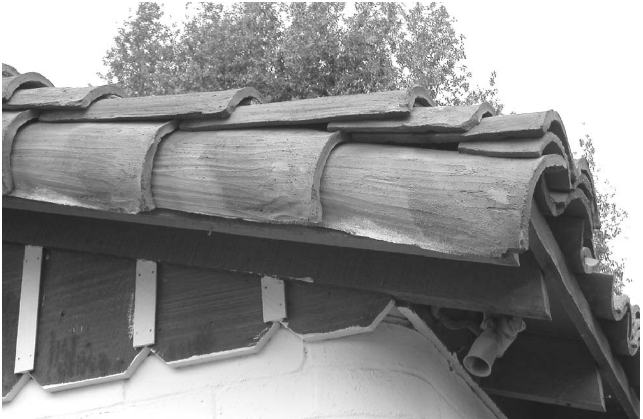
Detail view of tile at rake, 04/03
