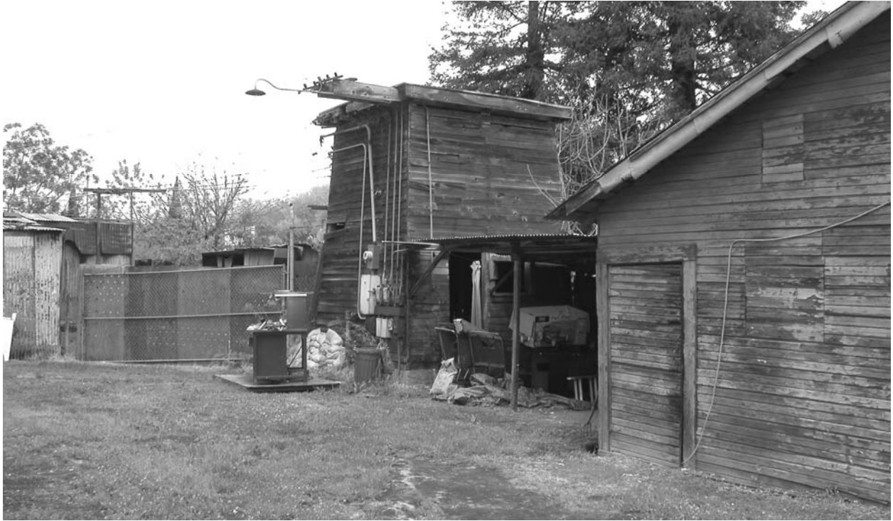
Tankhouse viewed from the south, 04/03
