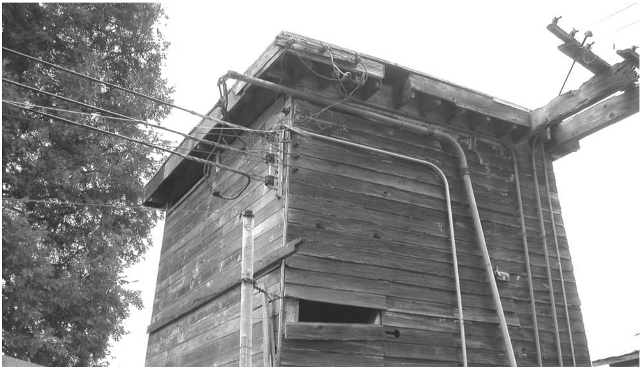
Detail view of top of tank house viewed from the northwest, 04/03
