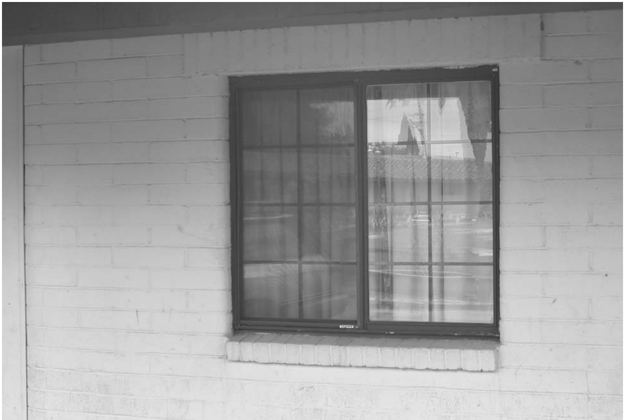
Retrofitted aluminum window in original motel unit, 04/03
