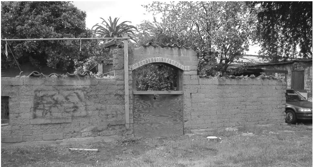
View from east of rear office patio fence, 04/03
