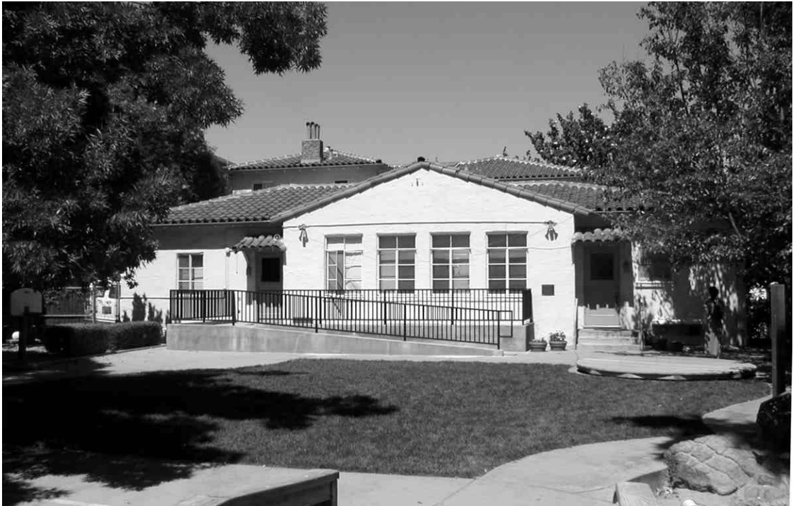
View of rear of building / F.Maggi, July 9, 2002
